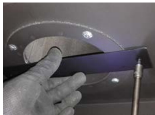
Figure 8.b.c Restrictor plate Installation
