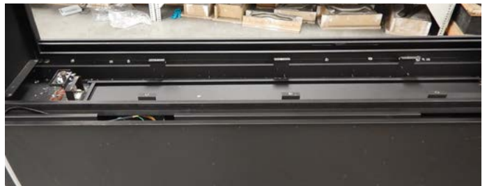
Figure 12.e Removing the Burner
