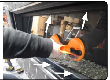
Figure 21.b Installing the door
