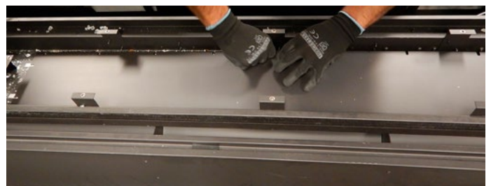
Figure 12.g Removing metal plate
