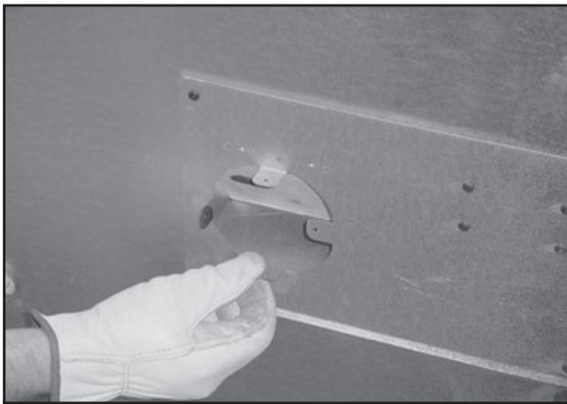
Figure 3.19 Bending Tabs on Outside Air Kit Collar
