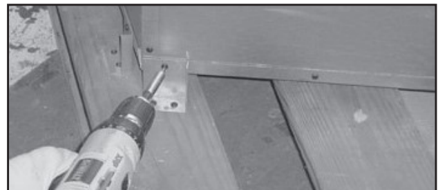
Figure 3.11 Removing Shipping Brackets
