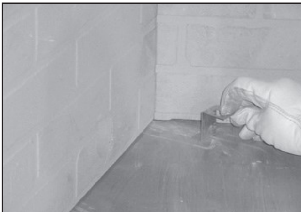
Figure 8.7 Slide Grate Retaining Bracket into Notch
