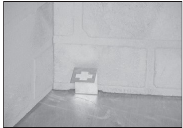
Figure 8.8 Grate Retaining Bracket in Place
