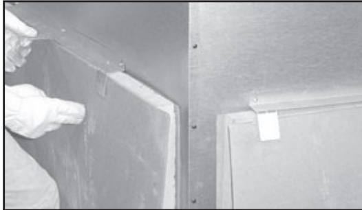
Figure 3.6 Unpack Back Refractory
