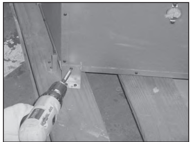
Figure 3.12 Removing Shipping Brackets
