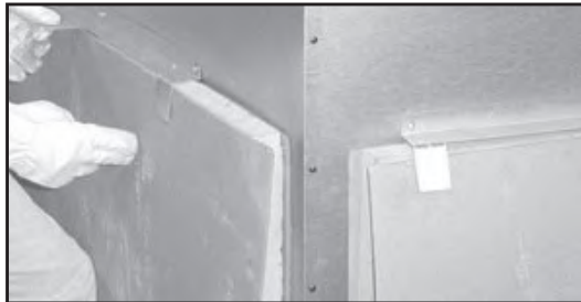
Figure 3.6 Unpacking Back Refractory
