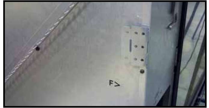
Figure 6.4 Side Nailing Tab in Shipping Position
