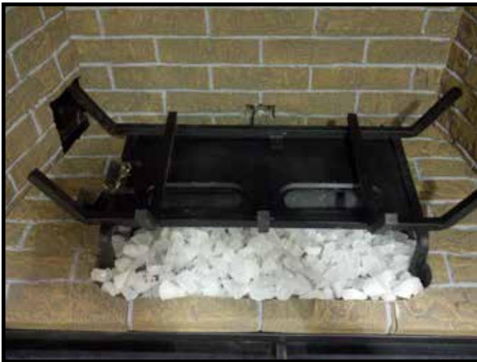
Figure 11.20. Ember Glass Area Covered with Teco-Sil
