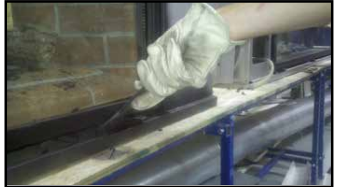
Figure 11.3. Inserting Glass Clip Tool
