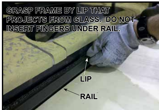
Figure 11.6. Installing Glass
