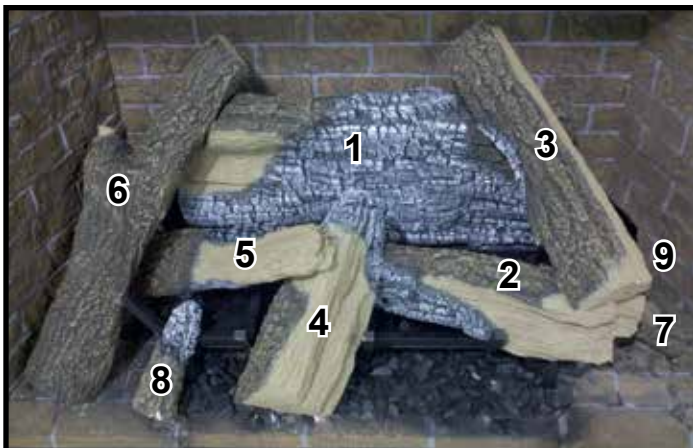
Figure 15. Log Set Installed (Log #9 not visible in this view).
