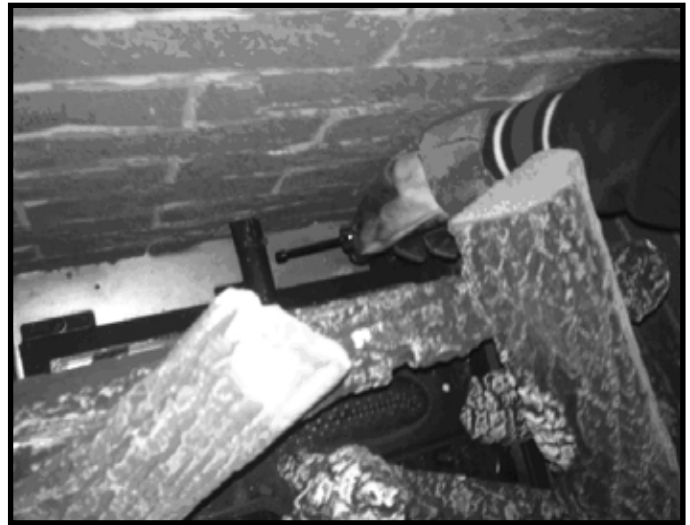
Figure 1. Air Shutter Location
