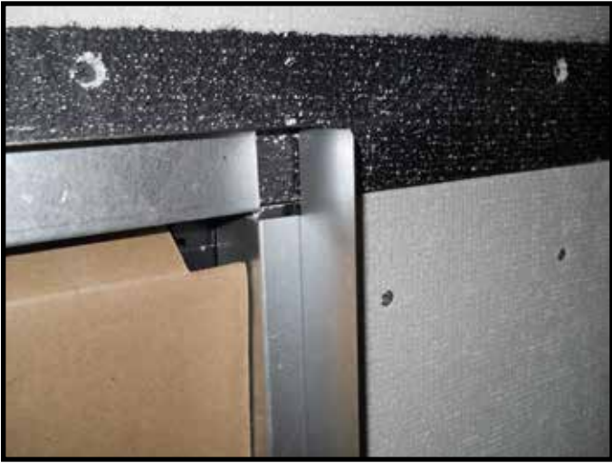
Figure 10.5 Finishing Template Bends
