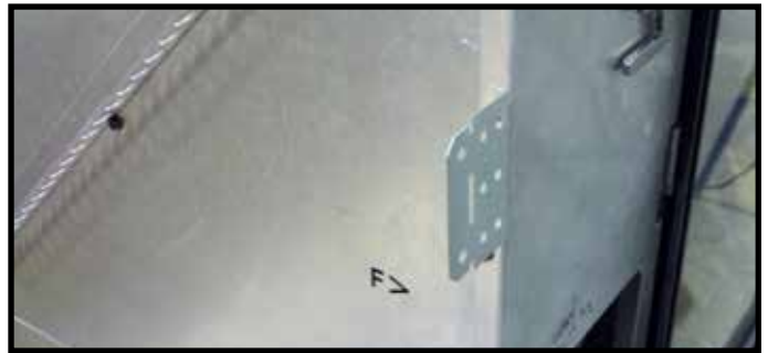
Figure 6.5 Nailing Tab Bent Out for Installation
