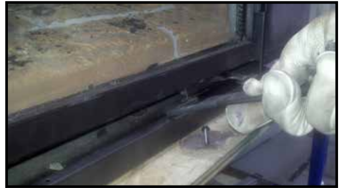
Figure 11.2. Glass Clip Tool Location
